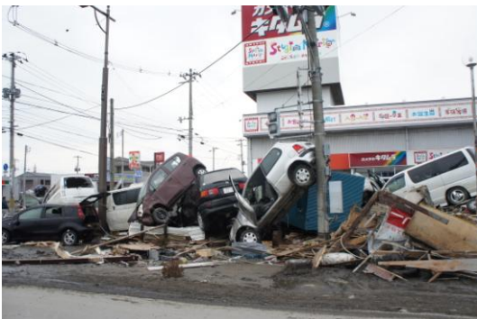
<Tsunami damage in Ishinomaki City>
